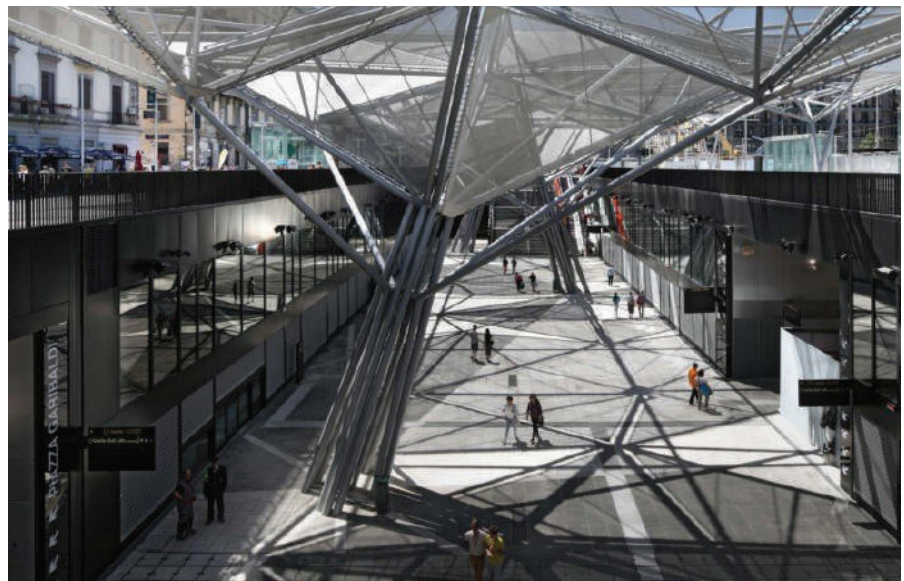
LOW CARBON DESIGN ILLUSTRATION UTILISING SUNLIGHT AS A NATURAL LIGHTING SOURCE AT PIAZZA GARIBOLDI STATION IN NAPLES, ITALY
