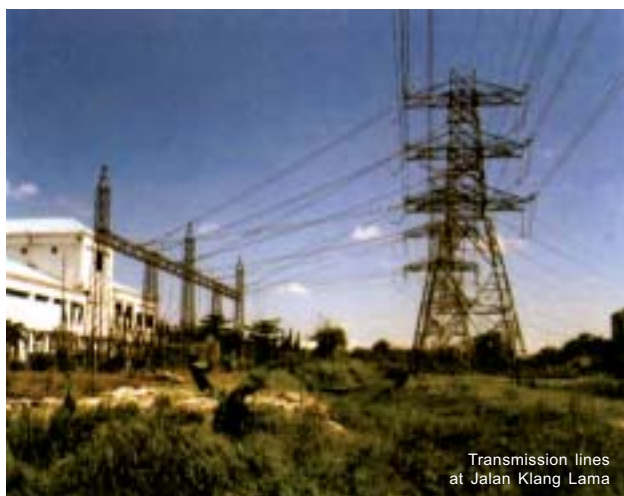
Photo 11.4: The national grid operates at 275kV and 132 kV.
